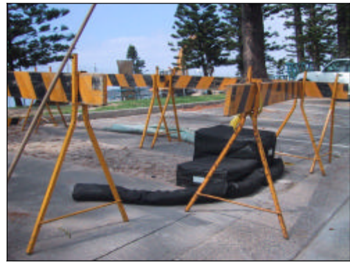
FilterBales & socks preventing sediment run-off from construction site
